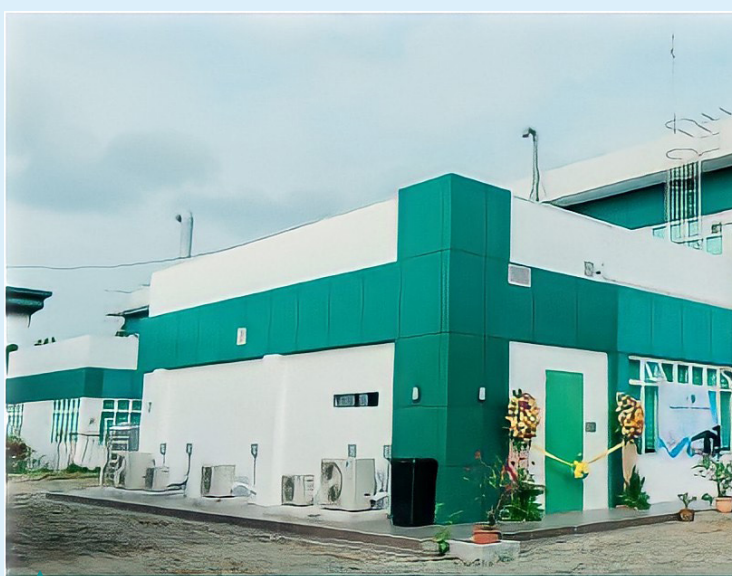
▲ An Anthrax Reference Laboratory located in Tuguegarao City, Cagayan. Photo taken by Black and Veatch Special Projects Corp.
