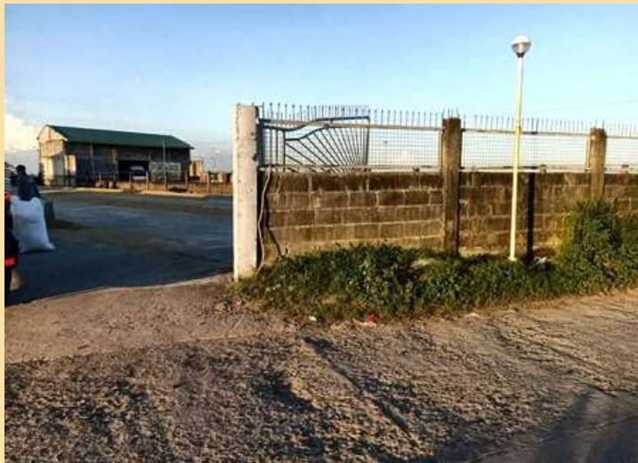
Image 4. Warehouse constructed where network road is accessible (Source: Gomez, 2021)
