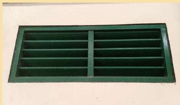
Image 11. Warehouse ventilation window (Source: Gomez, 2021)
