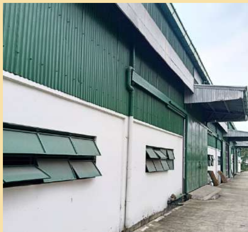
Image 13. Warehouse ventilation windows (Source: Gomez, 2021)
