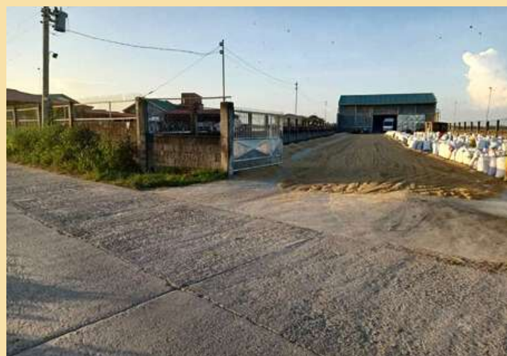
Image 5. Warehouse constructed where network road is accessible (Source: Gomez, 2021)
