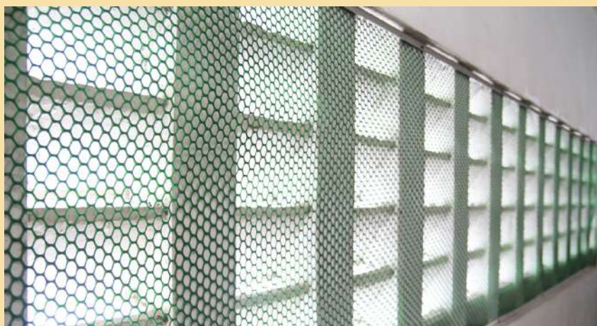
Image 22. Warehouse window with mesh screen (Photo taken at NFA ACA warehouse)
