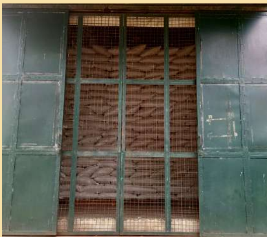
Image 20. Warehouse opening or doorway with mesh screens (Source: Gomez, 2021)
