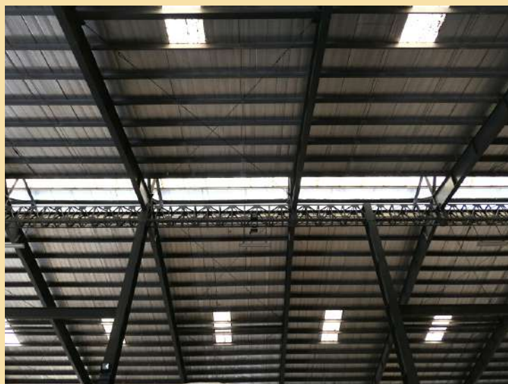
Image 26. Warehouse roofs (Photo taken at NFA ACA warehouse)
