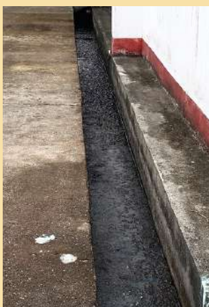
Image 14. Drainage around the warehouse (Source: NFA Region XI, 2019)
