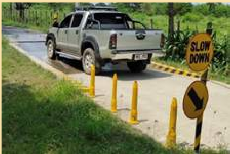
Image 14. Tire bath at the entrance point of Alsons Aquaculture Corp., Sarangani (Source: S. Mamalangkap. n.d)
