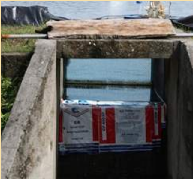
Image 32. Entrance gates for the water supply (Source: C. Lopez. n.d)
