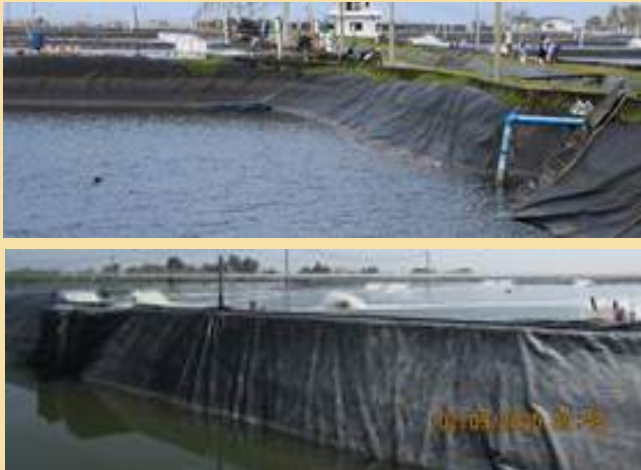
Image 10. Water dikes (Source: G. Coloma. n.d)
