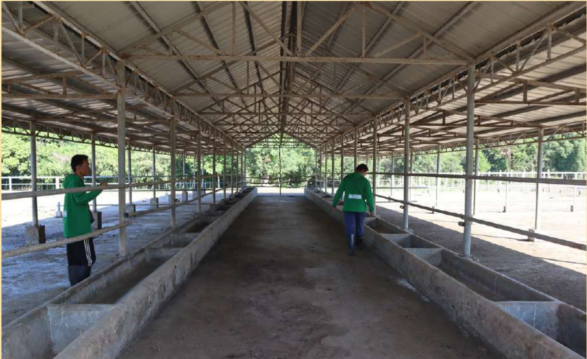
Image 26b. Personnel assessing the cleanliness of the facilities
