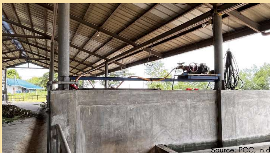
Image 23a. Well-elevated and properly maintained roof
