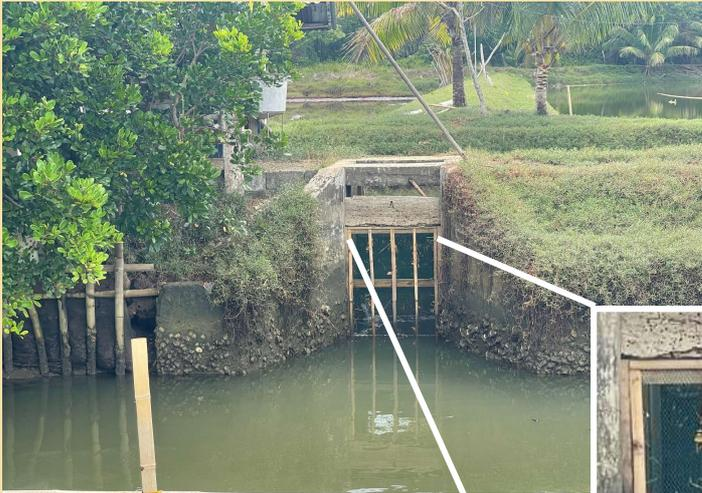
*Image 16a.* Pond gate with screen to filter incoming and outgoing water for earthen ponds
