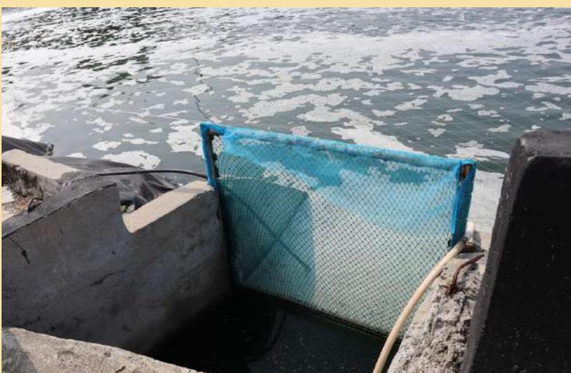
Image 32b. **Pond gate installed with screen**
