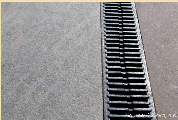
Image 42. Clean drainage channel for an effective drainage system
