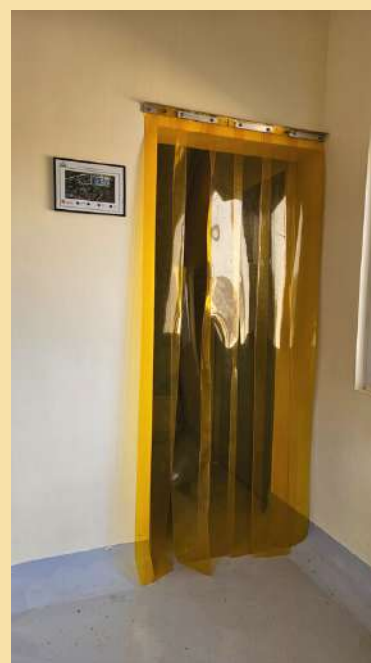
Image 51b. Packinghouse with plastic curtains or "fly curtain" to prevent entry of insects
